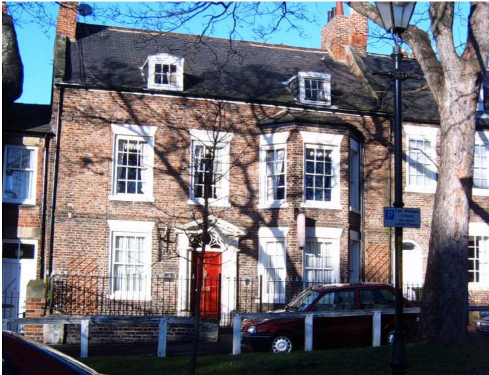
VIEW OF EXISTING SOUTHEAST ELEVATION- ELEGANT GEORGIAN FRONTAGE ONTO WESTOE VILLAGE
